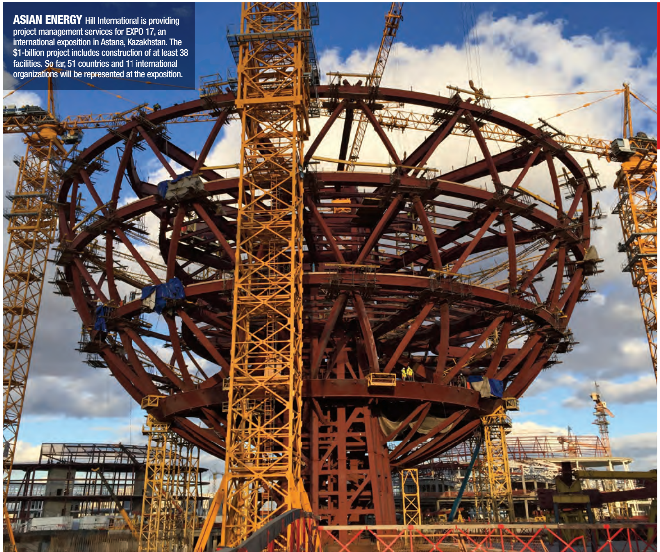
PHOTO COURTESY OF HILL INTERNATIONAL
